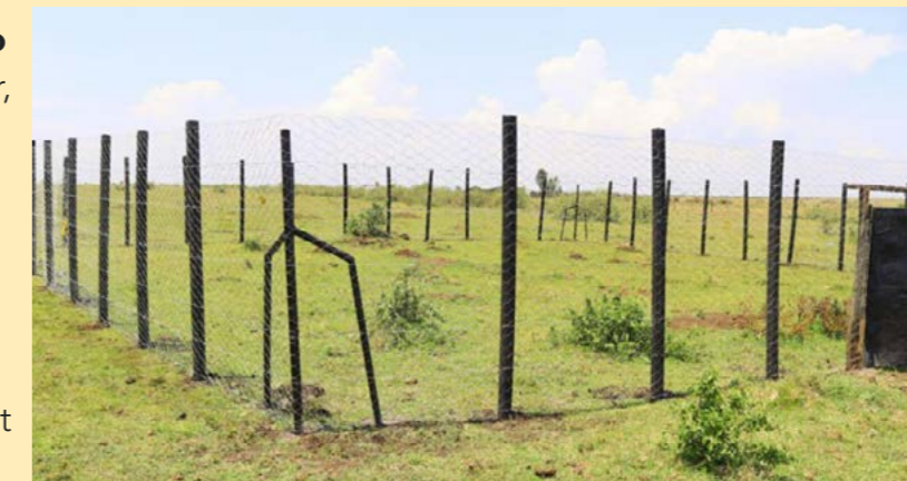
The newly constructed predator proof Boma for Mzee Mpooya of Olesere
