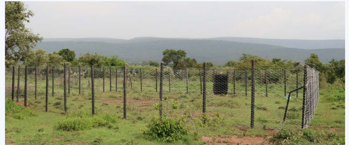
Figure 14: A newly constructed recycled plastic poles boma which is predator proof
