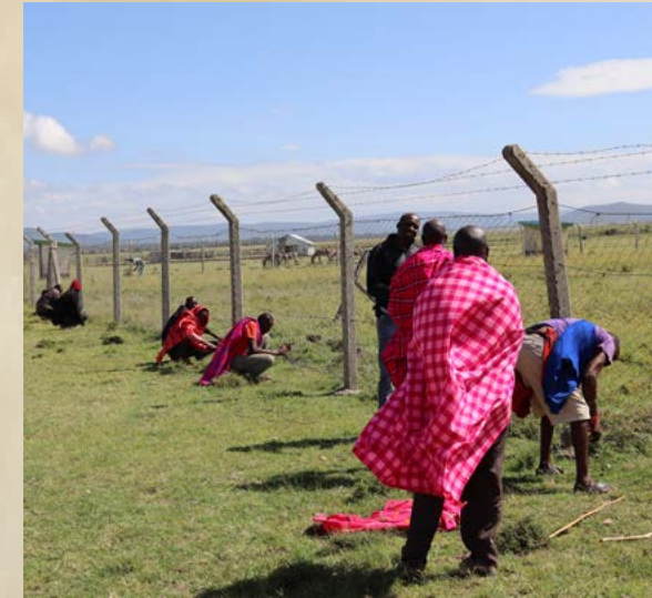
Community members volunteer to repair holes in the fence to prevent goats from destroying trees
