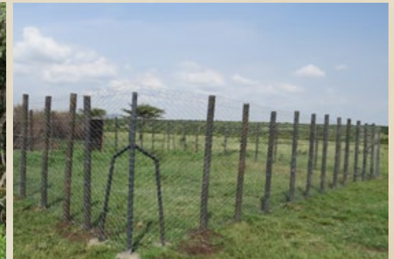
Figure 16. A completed recycled plastic poles boma at Enkeju enkoirien closer to Motorogi Conservancy
